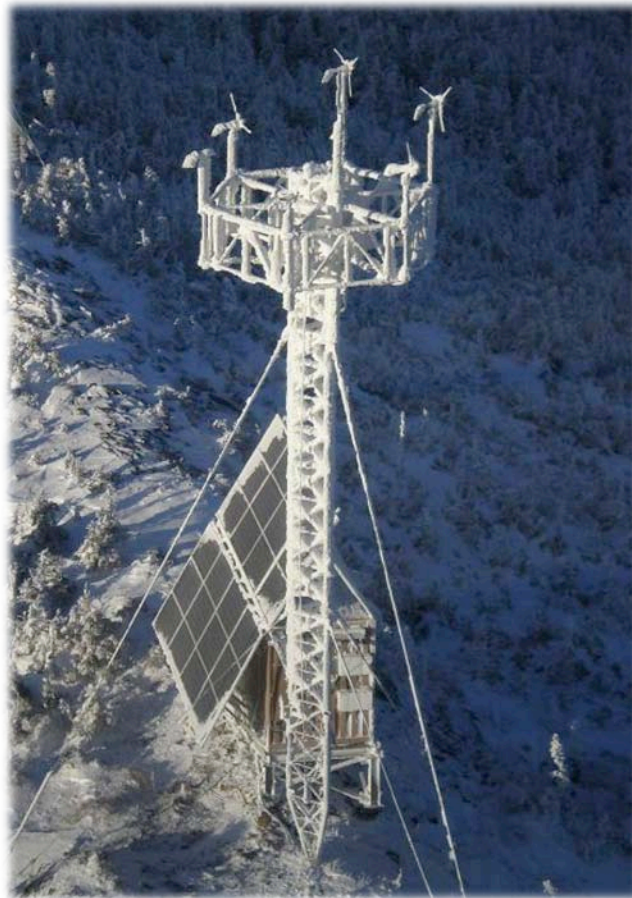
Figure 3: The rigged abilities of the SkyBuilt SkyStation to power a communication site in extreme environmental conditions. NOTE: This figure is shown for illustrative purposes only; actual installed equipment and system configuration may vary.
